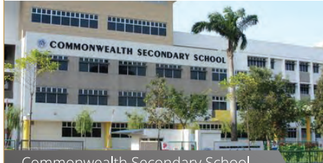
Commonwealth Secondary School
